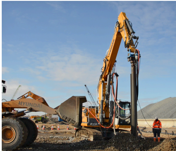
TE1 Top Feed rig (left) and BC1 Bottom Feed rig (right) with B27 vibroflots
