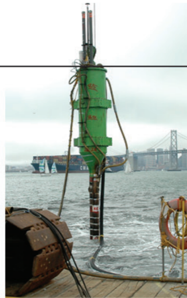
Conventional double lock rig with more than 7m high pressure chambers
