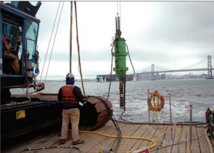
The rig was equipped with D-GPS and Gyroscope navigation tools to assure the correct location of stone column positions in over 30 m of water.
