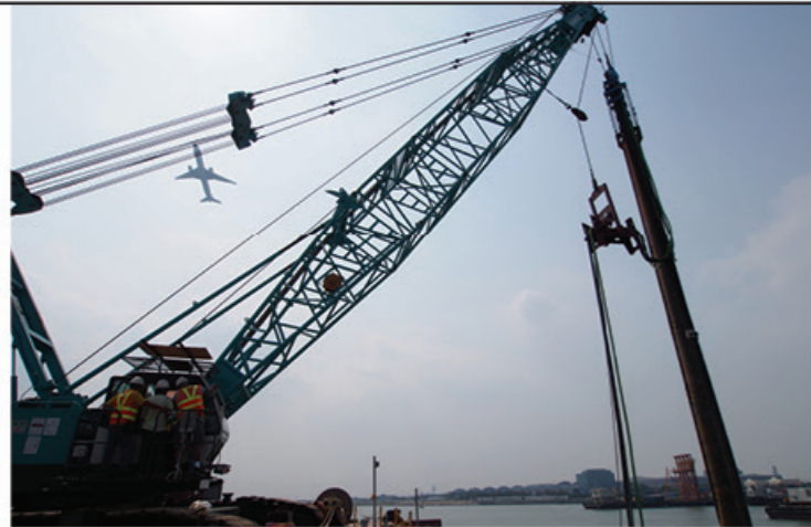
Offshore double lock low headroom rig with in soil submersible pressure chambers.
