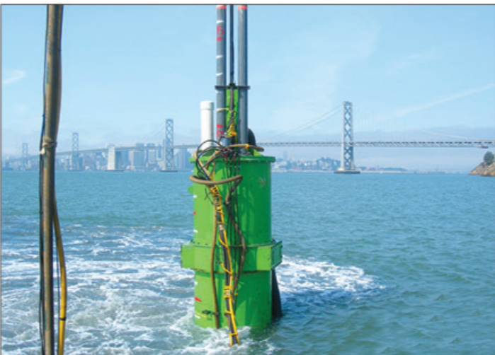
The rig was equipped with D-GPS and Gyroscope navigation tools to assure the correct location of stone column positions in over 30 m of water.
