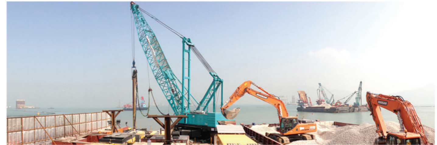
Barge setup with Gravel pumps, stone barge and another double-rig barge in the background
